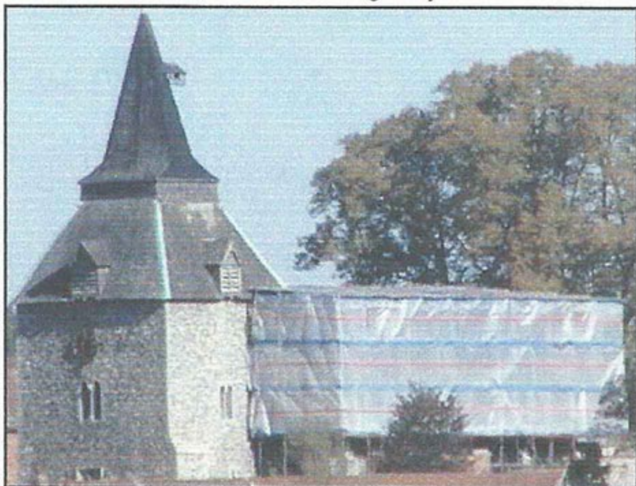
Sheeting covering the South side of the Church.
